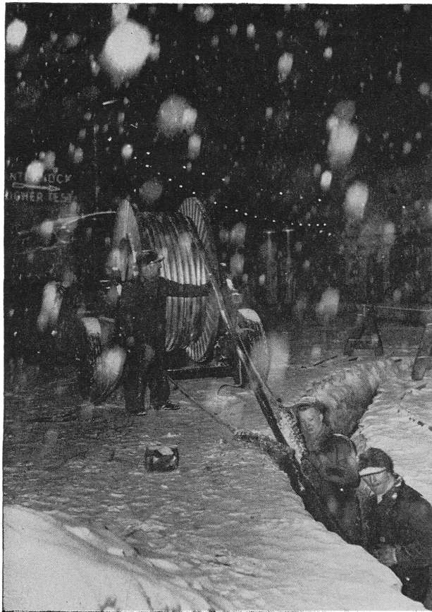
IN 5° COLD a new cable is laid in a River Grove lumberyard for the new office. The equipment for it left a New Jersey factory a few hours after the fire.
