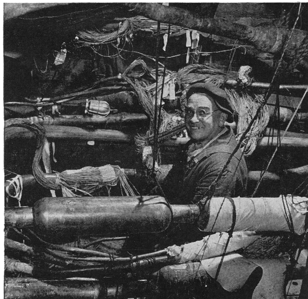
1,400 WIRES in one of main cables are spliced separately and by hand. This was probably the most exasperating repair job of all those that had to be done.
